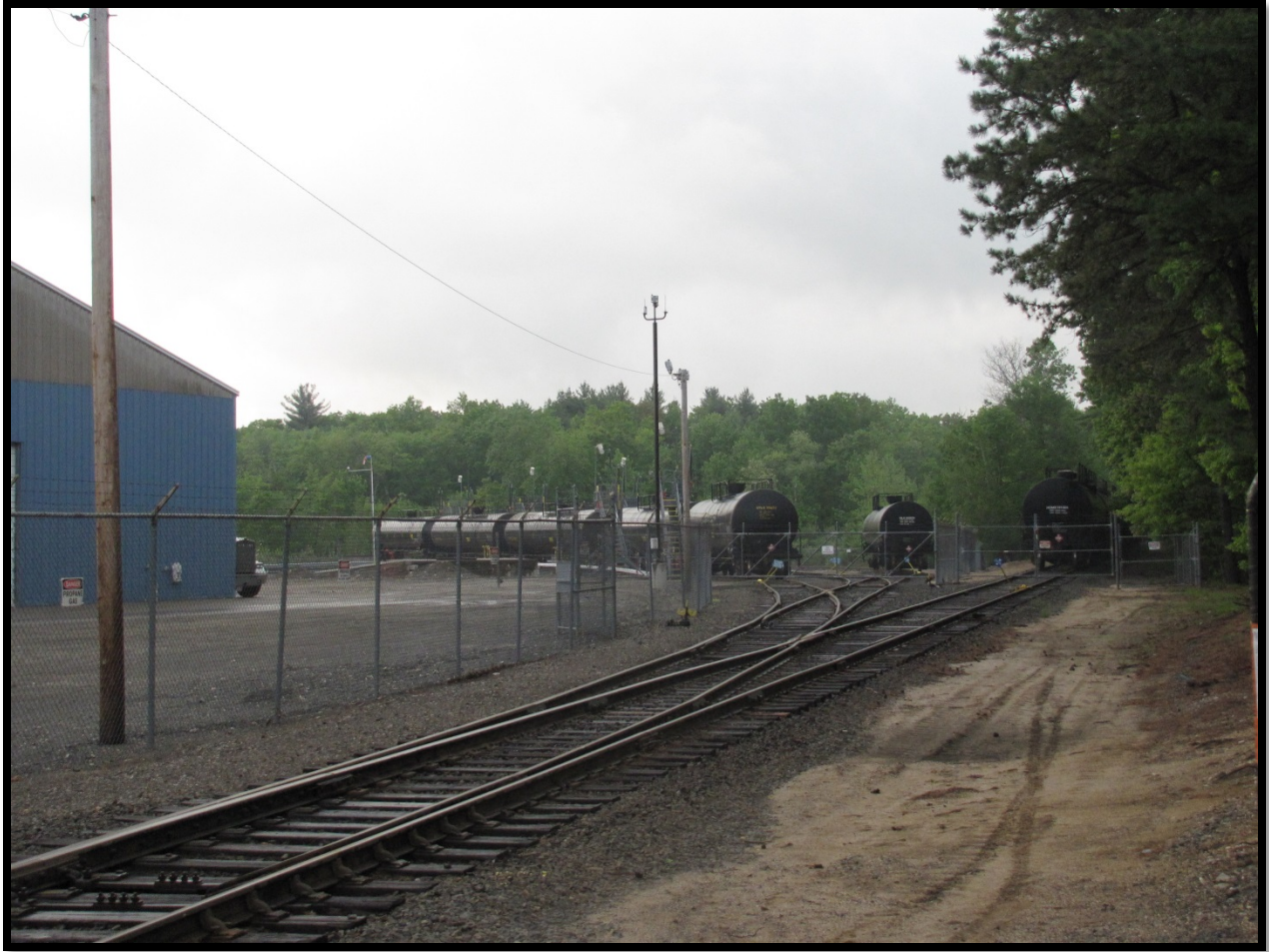
Figure 13: Pioneer Valley Railroad Propane Transload Facility. Westfield, MA (2014)
