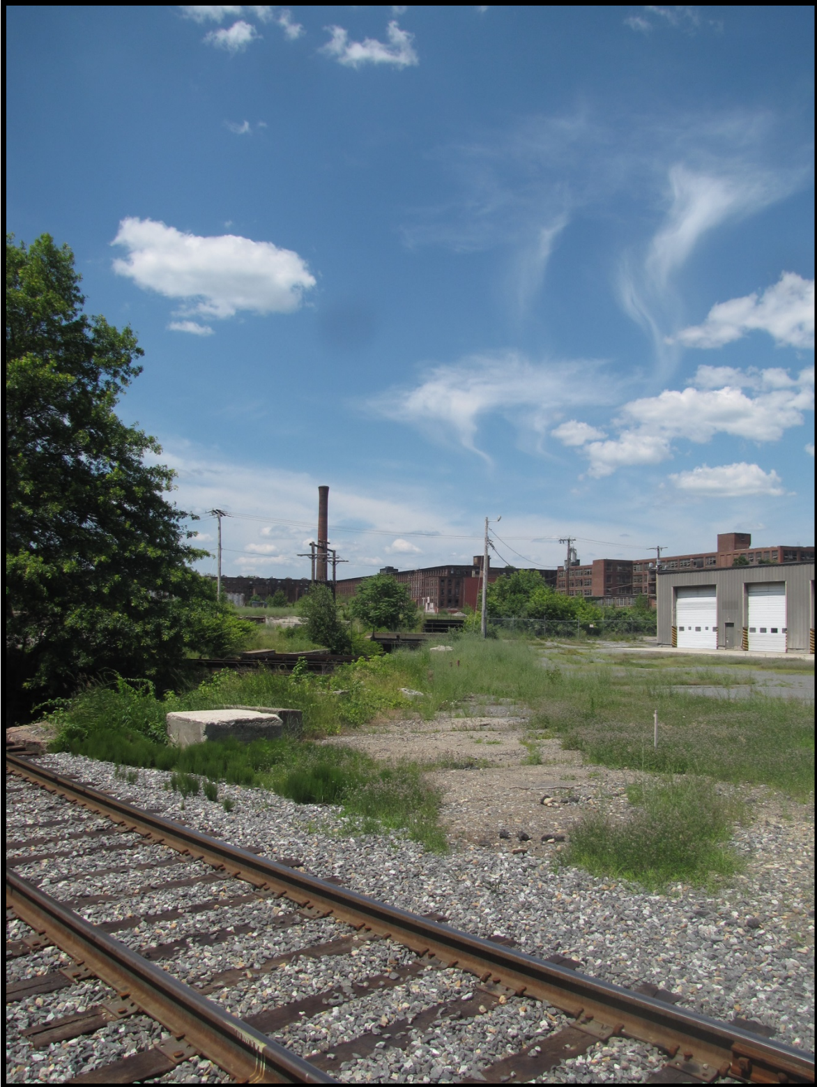
Figure 6: Grafton & Upton Railroad's Repaired Line, Draper Mills. Hopedale, MA (2014)
