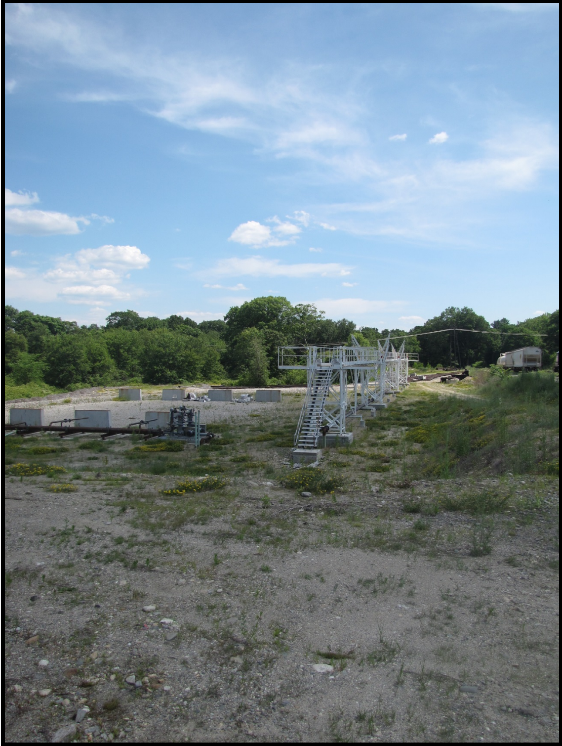
Figure 4: Grafton & Upton Yard, Construction of Propane Transload Facility, Grafton, MA (2014)
