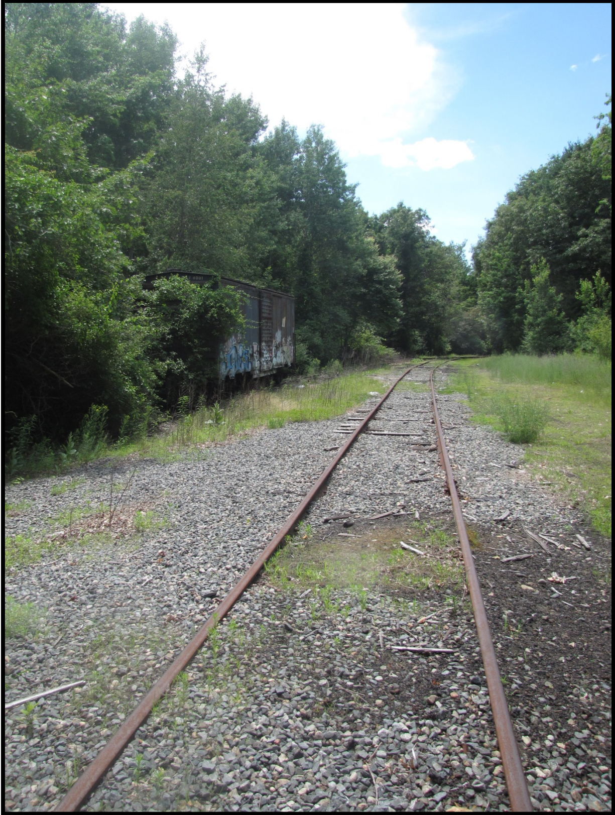
Figure 4: Bay Colony Railroad's Millis Branch, looking West. Millis, MA (2014)
