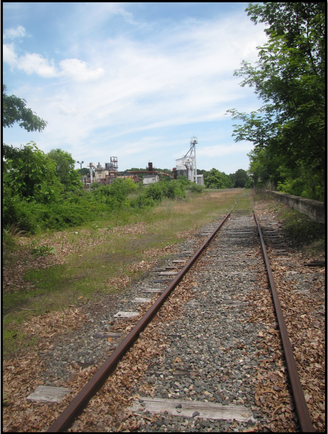
Figure 3: Bay Colony Railroad's Millis Yard, Former GAF Shingle Factory. Millis, MA (2014)
