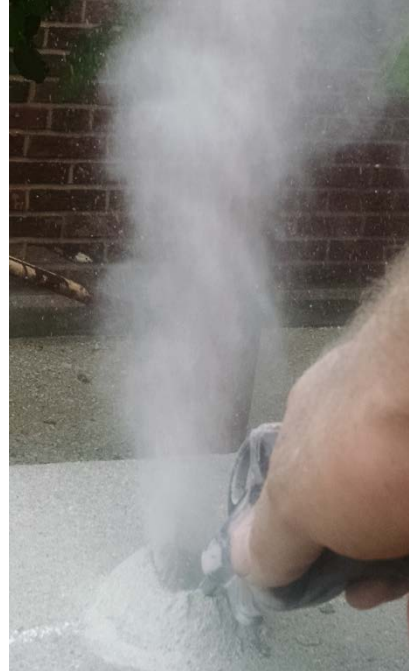
Figure 8.3 Hole Cleaning with Compressed Air
