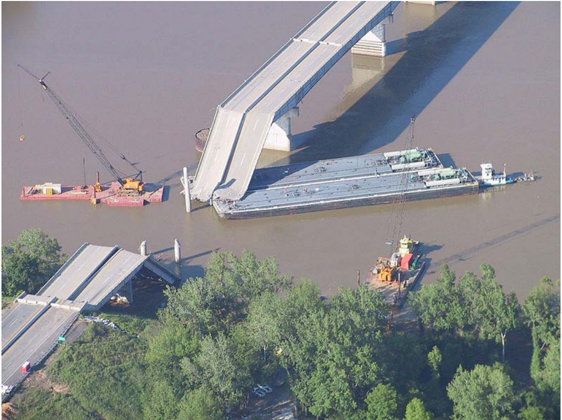
Figure 1.5 Barge collision with I-40 Bridge in Oklahoma ( http://en.wikipedia.org/wiki/I-40_bridge_disaster )
