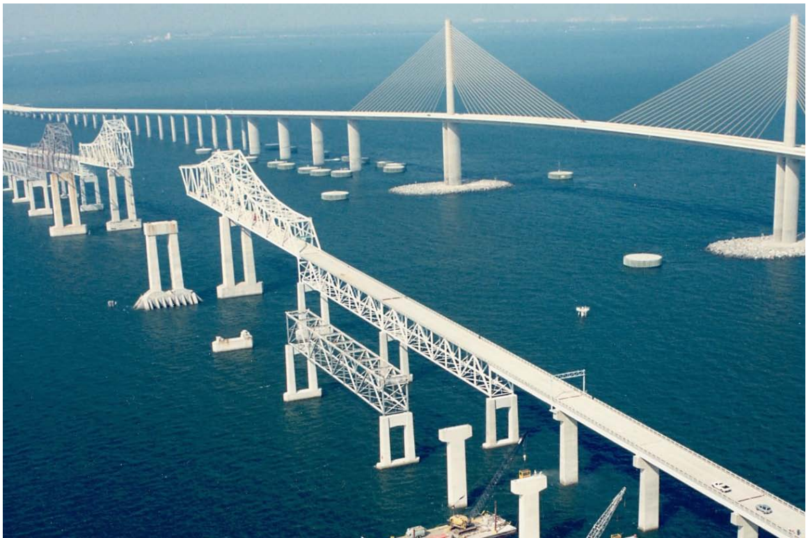
Figure 4.8 Old Sunshine Skyway Bridge (front) with replacement (back)
