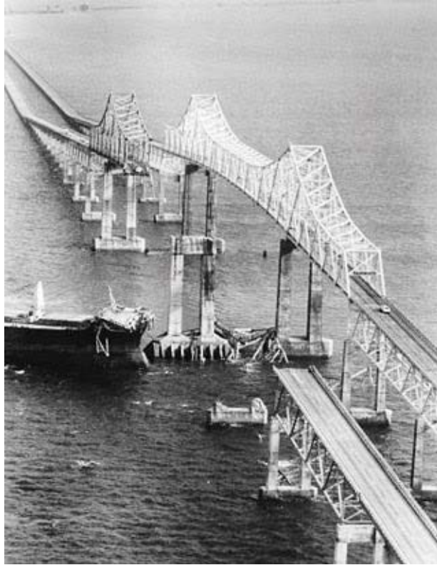
Figure 1.3 Disaster of the collapse of the Sunrise Skyway Bridge ( http://www.panoramio.com/photo/53278080 )
