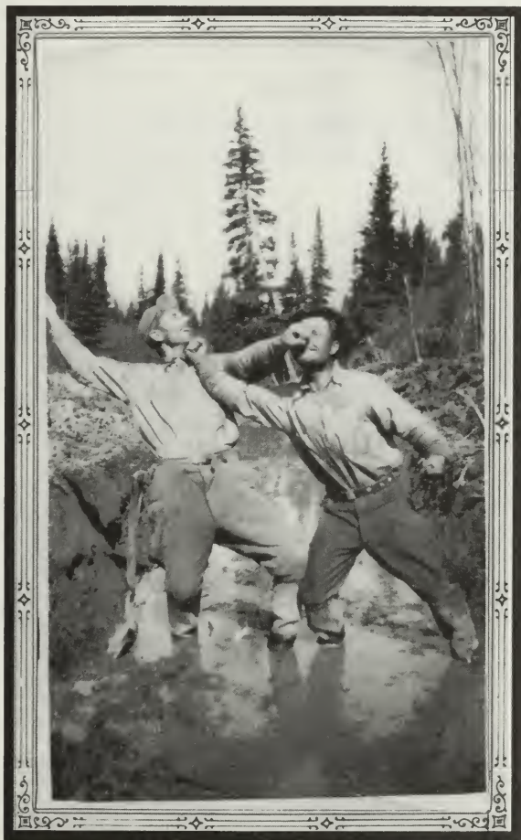
Harry Digging Ditches #5
