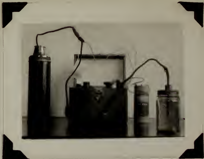
Plate 3. Thermocouple, potentiometer, and cold junction.
