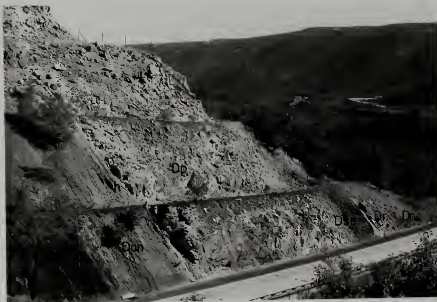
Figure 57.—Lehigh-Schuylkill facies of Onesquethaw Stage, Northeast Extension, Pennsylvania Turnpike, cut through Stony Ridge at West Bowmans, Carbon Co., Pa. (P22). The section ranges from Lower Devonian New Scotland chert (Dns, rubble at extreme right) to Middle Devonian Marcellus black shale (Dm, at left). The Ridgeley Sandstone (Dr), Schoharie-Esopus Formations, undivided (Dse), Palmerton Sandstone (Dp), and Onondaga Limestone (Don), with reddish Hazard Member (h) at base, are completely exposed.
