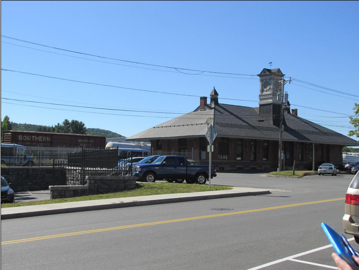
FIGURE 62: TRAIN STATION (EXISTING CONDITIONS)
