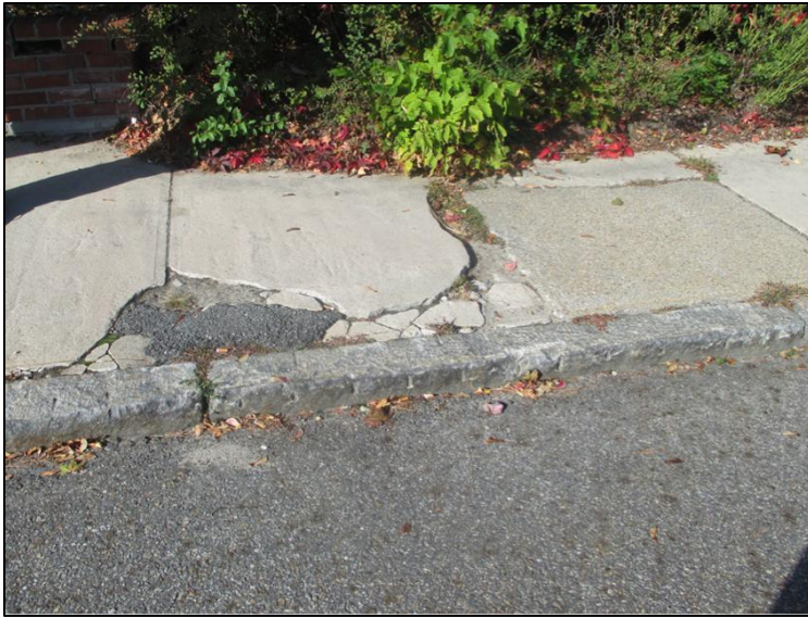
FIGURE 53: EXAMPLE OF EXISTING SIDEWALK CONDITIONS
