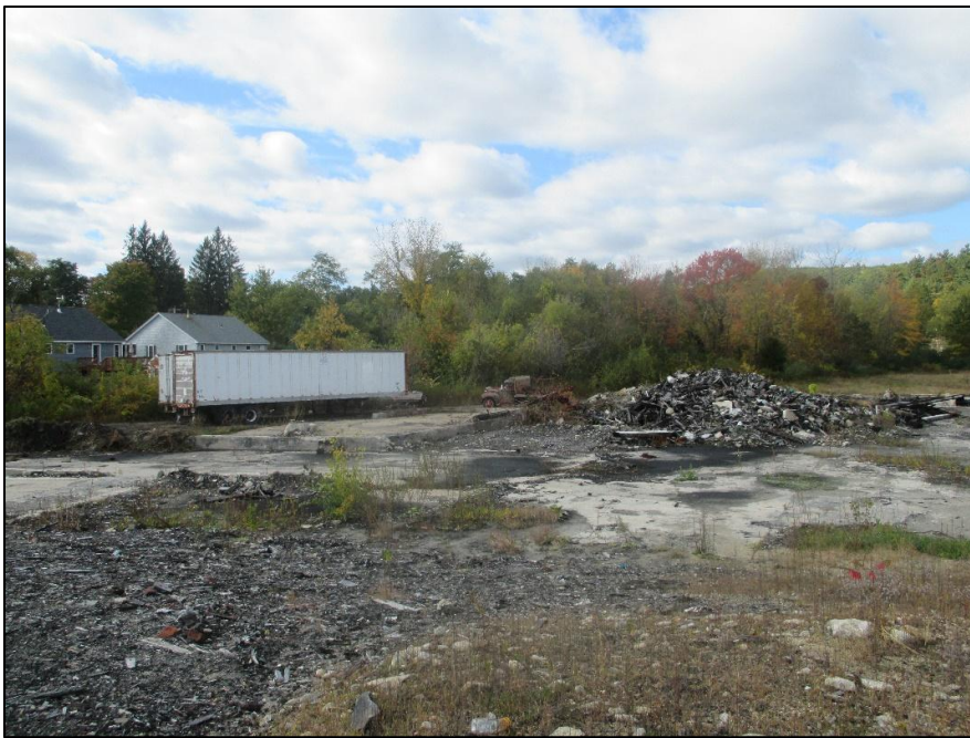
FIGURE 36: CASS FACTORY "GROUND ZERO," 2014
