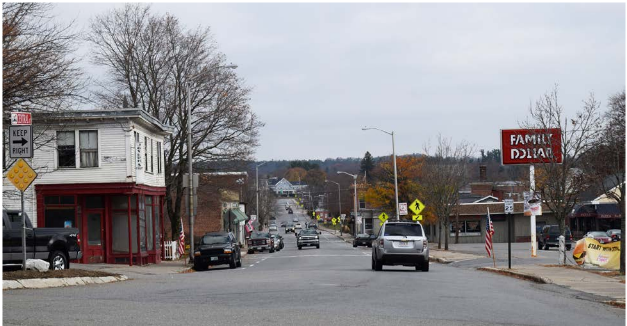
Top left: Blair Square, the ‘epicenter of town’ according to one Winchendon resident; Top right: Hungry4Pizza, once a popular downtown destination, closed recently, joining other vacancies on Central Street; Bottom: A view of Central Street corridor facing north from Blair Square.
