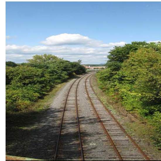
Railroad Corridor dissects the North End.
