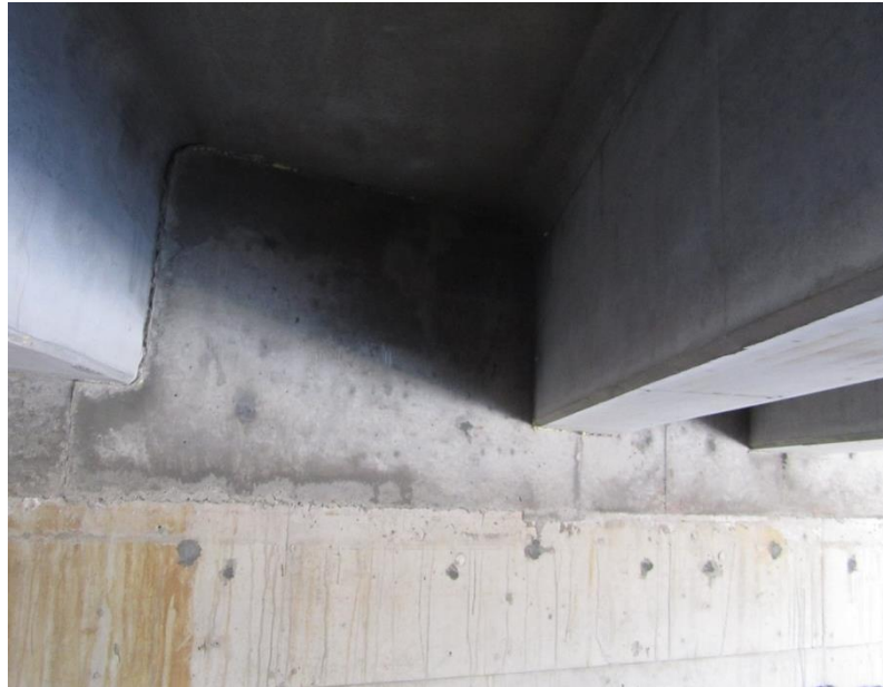
Figure 1-3: Full Integral Abutment after Construction
