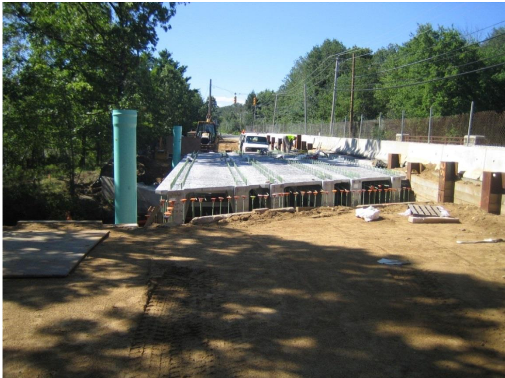
Figure 2-6: Beams 6, 5, and 4 Placed on the Abutments during Phase 1
