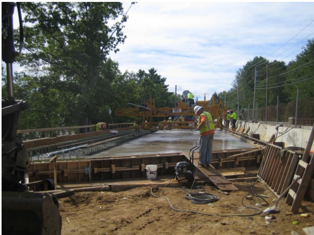
Figure 2-7: Casting the Concrete Deck (Phase 1)
