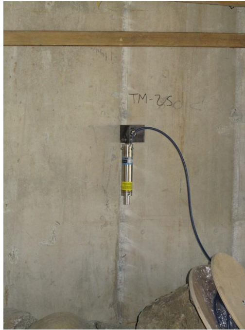
Figure 2-16: Tilt-meter Right after Being Installed
