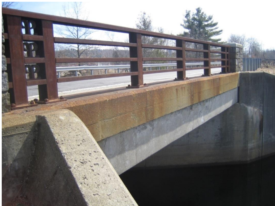
Figure 2-1: Existing Brimfield Bridge
