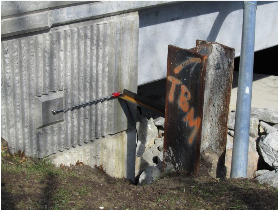
Figure 2-16: Picture of Crackmeter Installation on Abutment
