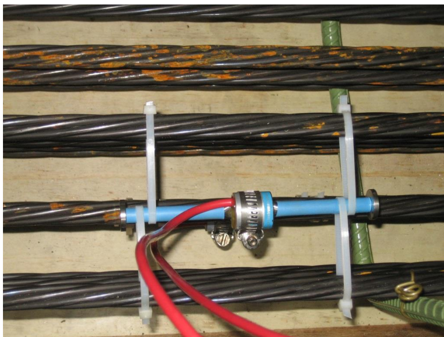
Figure 2-14: Longitudinal Strain Gauge Attached to Strands
