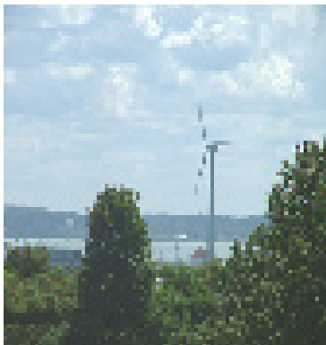
Wind Turbines at Hull
