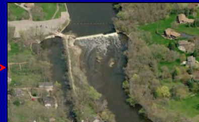
Mequon-Thiensville Dam Passive "Nature-Like" Fishway (2010)
