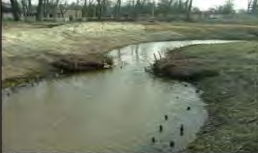
Pools above each rock weir, allowing fish to rest and continue swimming upstream
