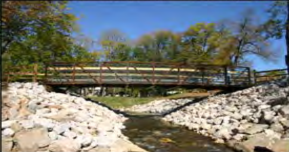
The fishway entrance and first rock weir, located beneath the pedestrian bridge
