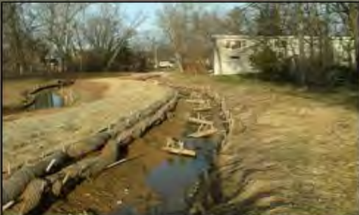
Submerged logs, placed during construction to provide overhead cover
