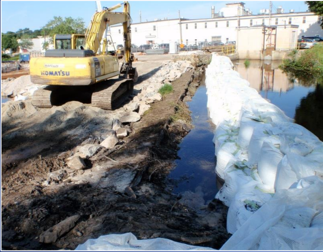
Upstream Super Sack Dam
