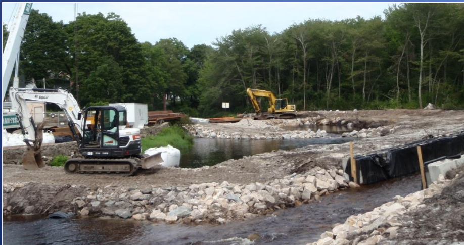
Downstream Temporary Dam
