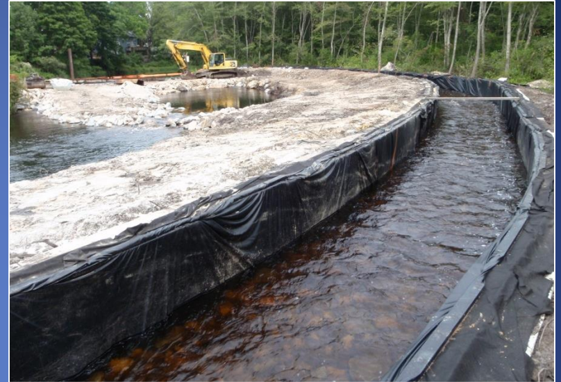
Temporary Flow Diversion Bypass
