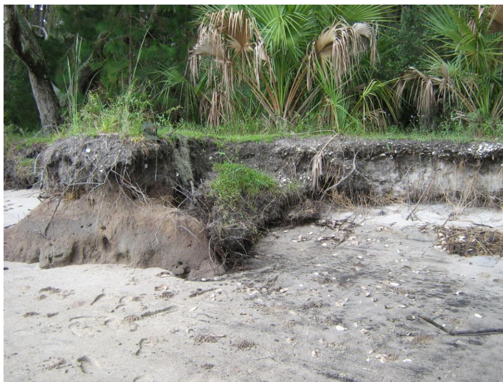
Figure 13. Brickhill bluff, erosion after heavy storm in 2007 (Courtesy John Fry, CUIS National Seashore).
