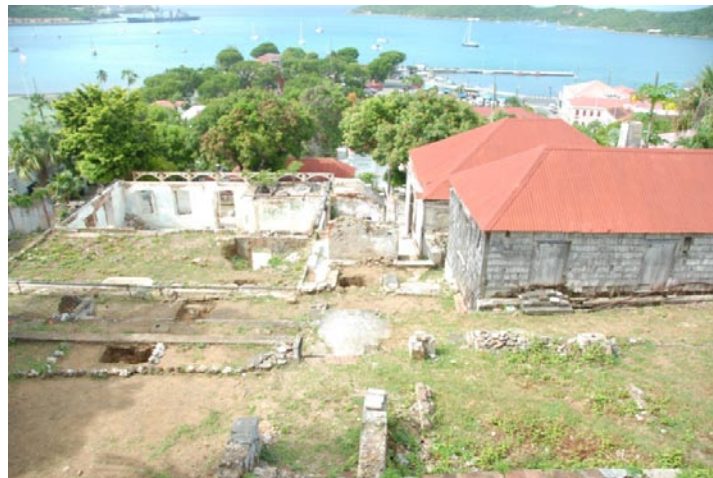
Figure 1. Ruins of main house at Magens House (left), servant quarter (earlier enslaved laborer quarters) and cook house (right).
