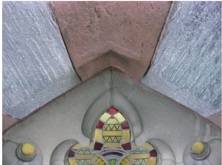
Figure 4.4. Stained glass and tracery. The most ornate glass pattern is at the top of each window; here as well can be seen the small, circular stained glass ornamentation that require precise measurement in the re-cast concrete tracery frame.
