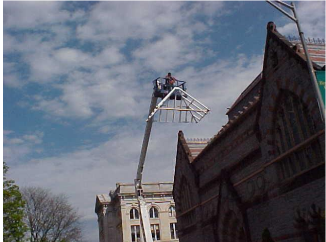
Figure 3.17. Removing the skylight in 2001. Photo, courtesy Ron Salice.
