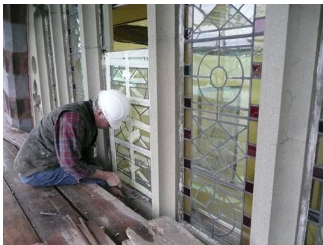
Figure 4.3. Removing the stained glass. Above, Chuck Woodard pulls out a storm window in order to document and then tape the panels. Below, David Guarducci chips at caulking holding the panel to the stone frames. Photos, the author.
