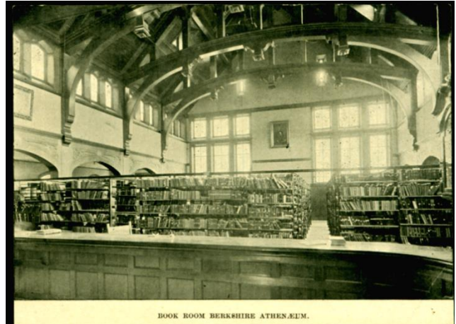
Figure 4. Cathedral-like ceiling of addition, with quartered oak trusses. Courtesy, Berkshire Athenaeum
