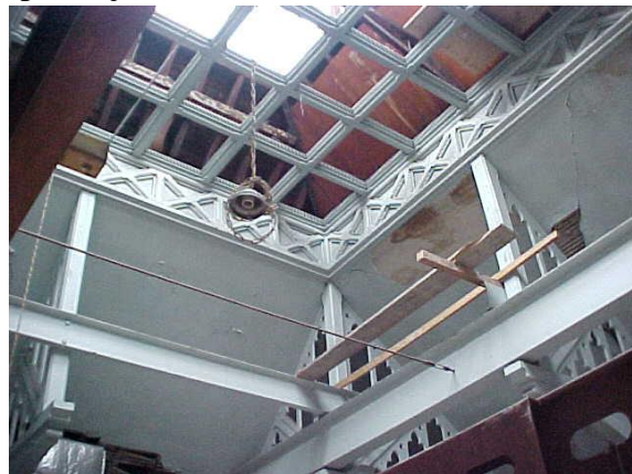
Figure 3.12. Original skylight and steel beams placed in 1945. With a suspended ceiling added in the 1978 renovations, the skylight is no longer visible. Photo, courtesy Ron Salice.
