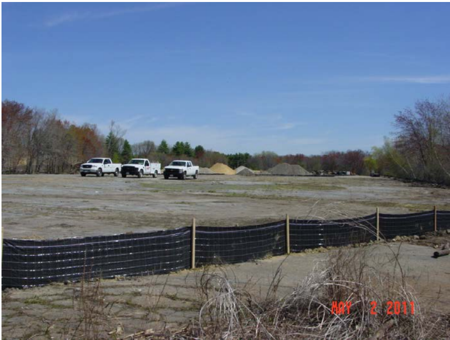
View of the parking area at Hartwell Farms
