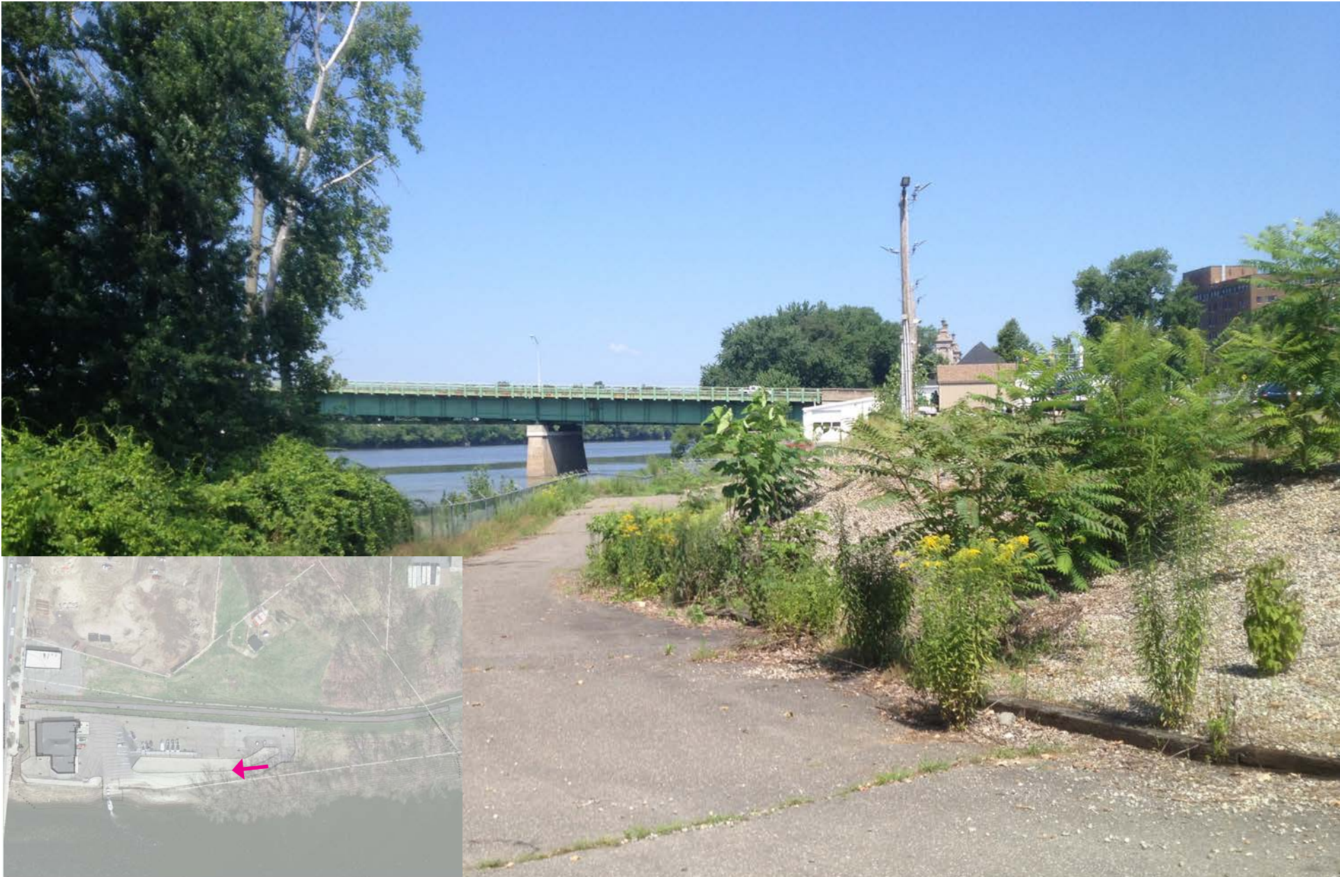
View of loop road looking north-west
