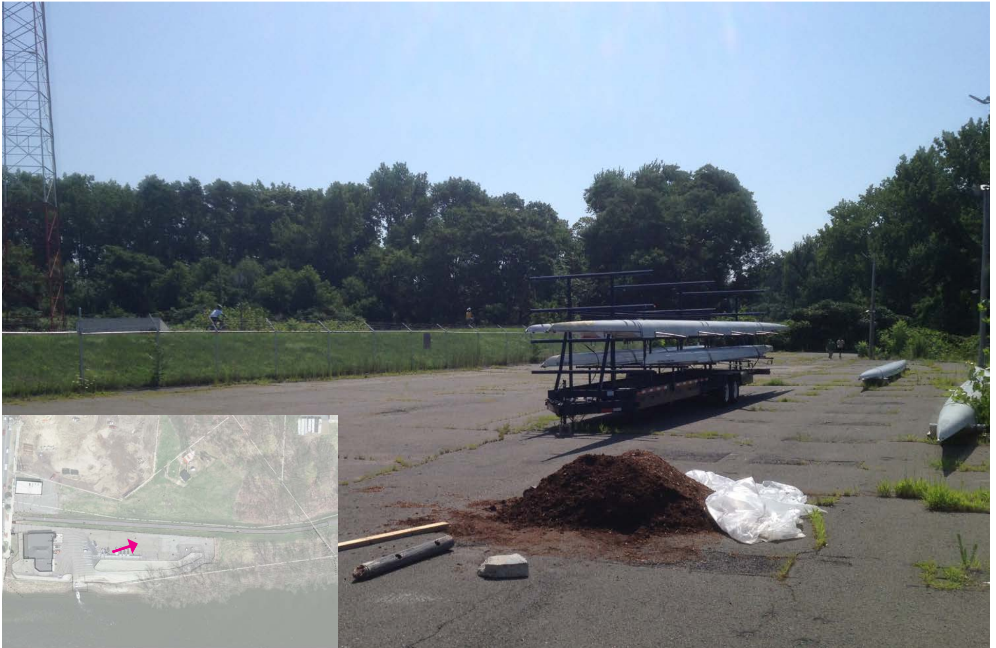
View of elevated fill area and flood levee/bike path in the background
