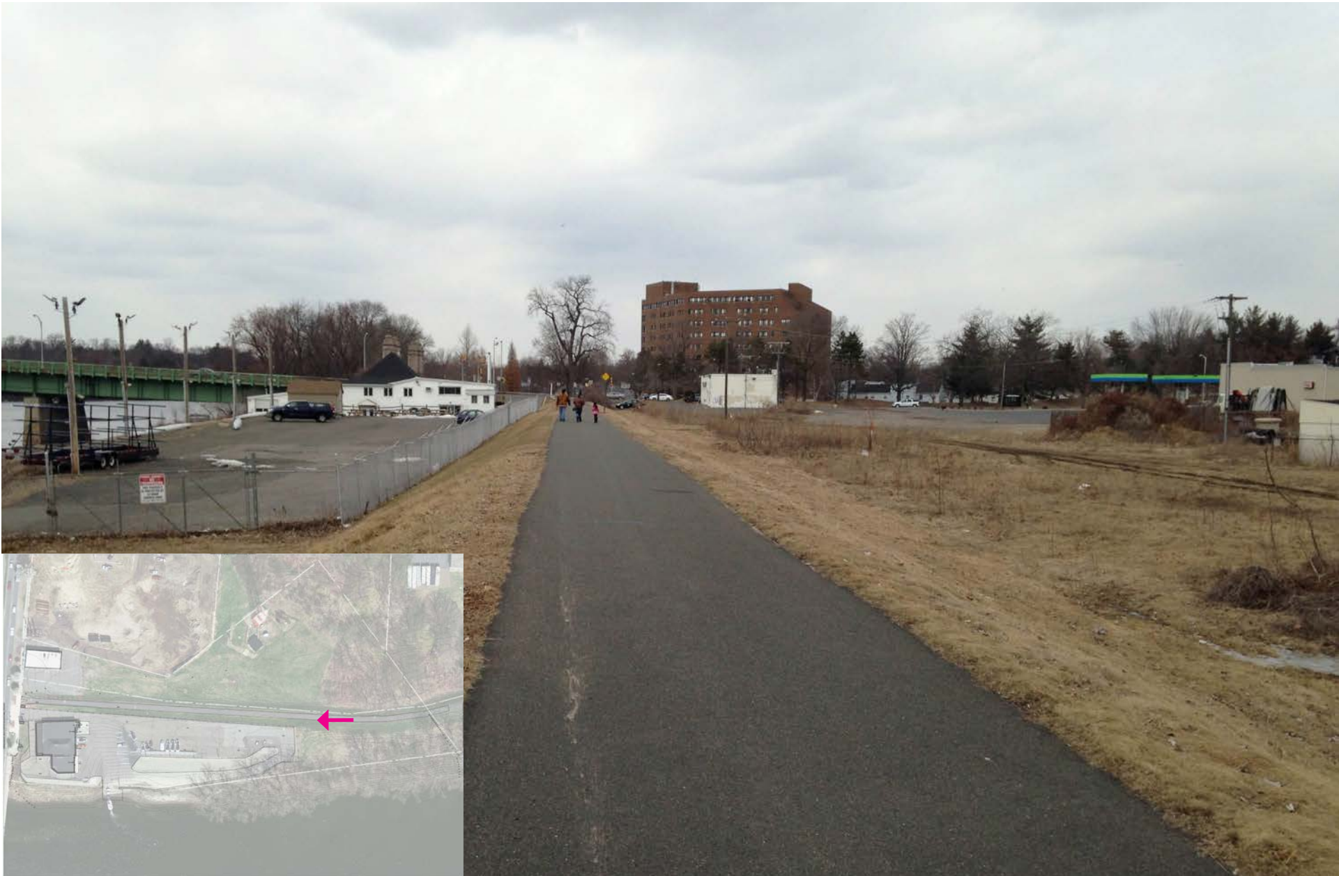
View on top of the flood wall looking north-west at the PVRC boathouse
