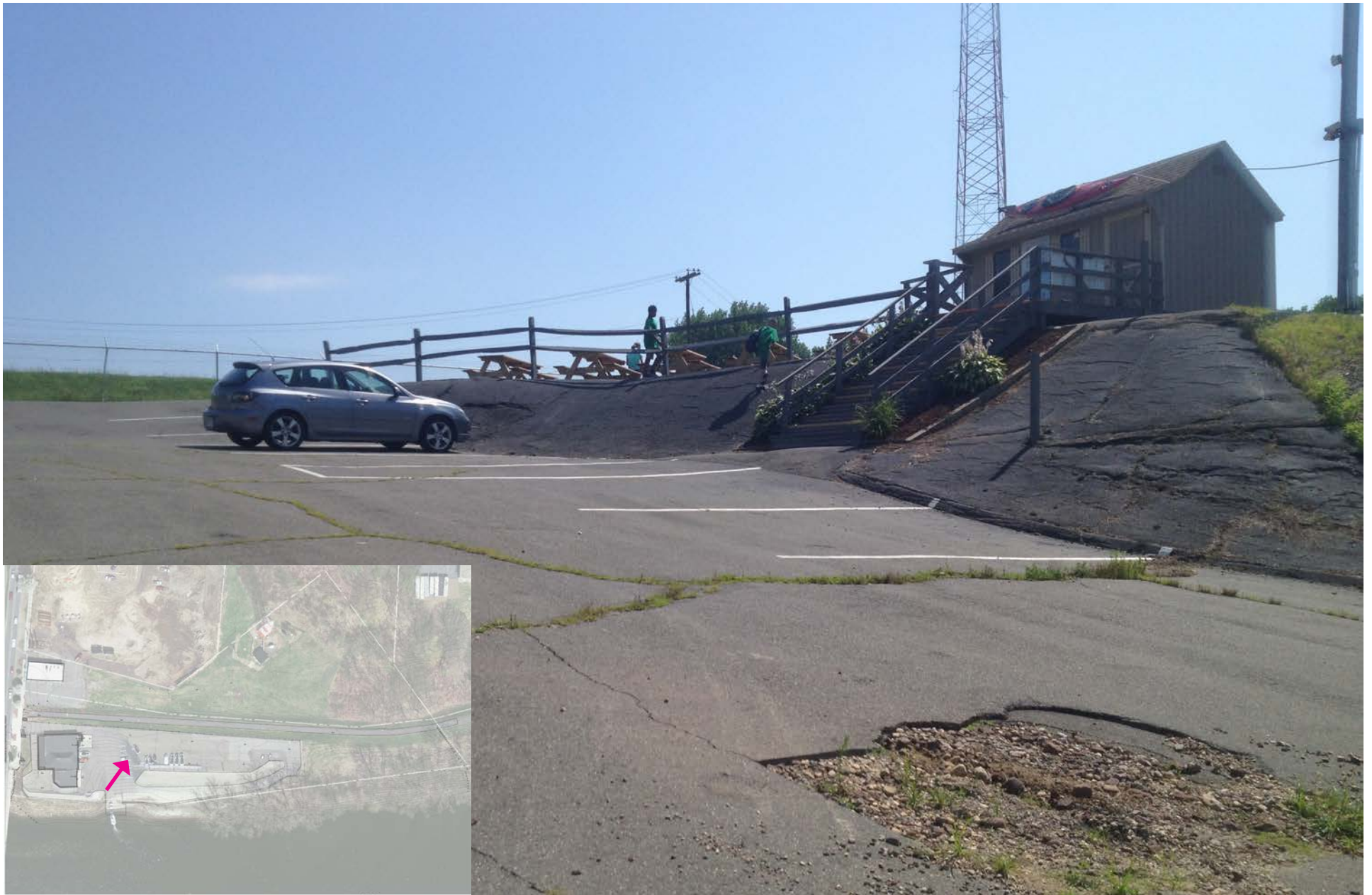
View looking up the boat ramp and the steep slope
