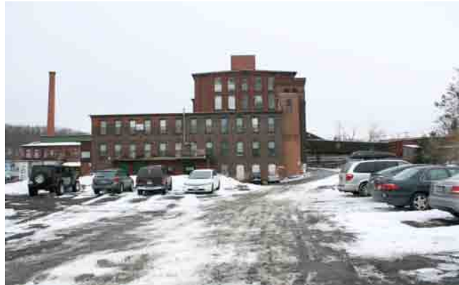
The Indian Orchard Mills are a cluster of historic buildings that serve diverse tenants.
