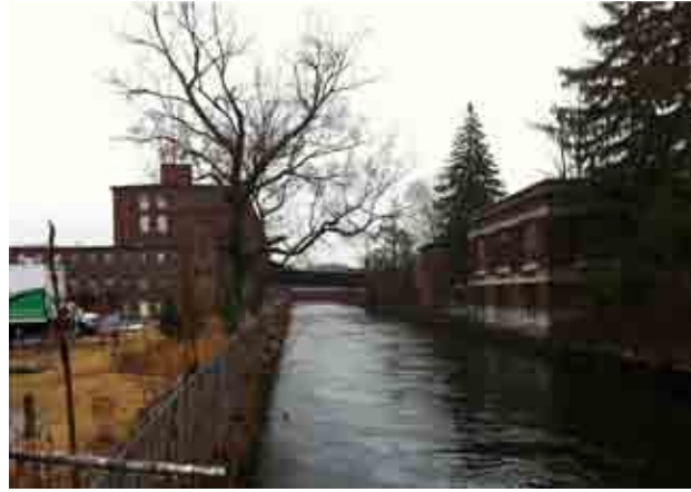
Existing conditions beside the Mill include a canal that is fenced off and has very little connection with people visiting the site.
