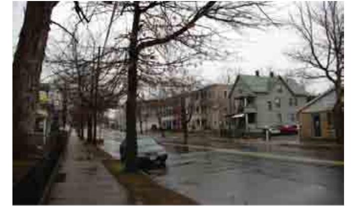
The Residential C District has a variety of housing styles and has some of the higher density housings.
