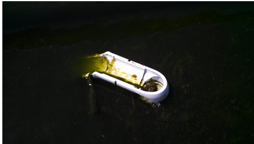
Figure 3-9: Areal view of a 2-inch ramped effluent standpipe submerged in a raceway pond at the AFS (Chang, 2014).
