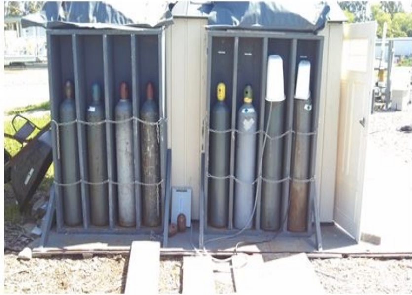
Figure 3-21: The 50-lb CO 2 tanks were secured in a housing unit at the AFS. One tank was used at time to release carbon dioxide into a specific pond with pH levels above the set limit (Chang, 2014).
