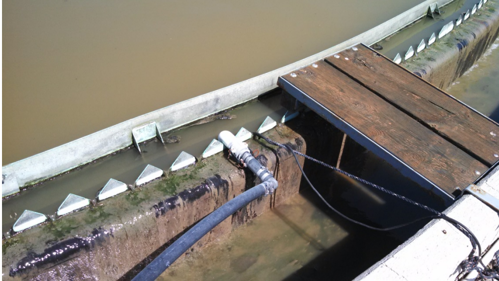
Figure 3-6: The Algae Field Station's source of clarified municipal wastewater was collected from the WRRF's Western primary clarifier, in between the overflow weir and scum baffle (Kraetsch 2015).
