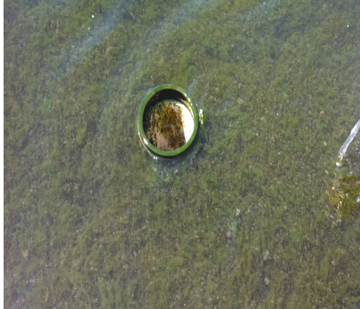
Figure 3-10: Areal view of a 4-inch vertical effluent standpipe submerged in a raceway pond at the AFS (Chang, 2014).
