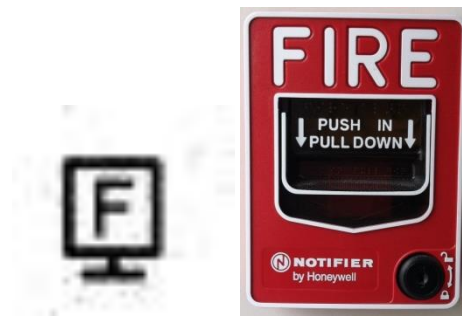
Figure 15 - Plan view symbol and photo of manual pull boxes within building.
