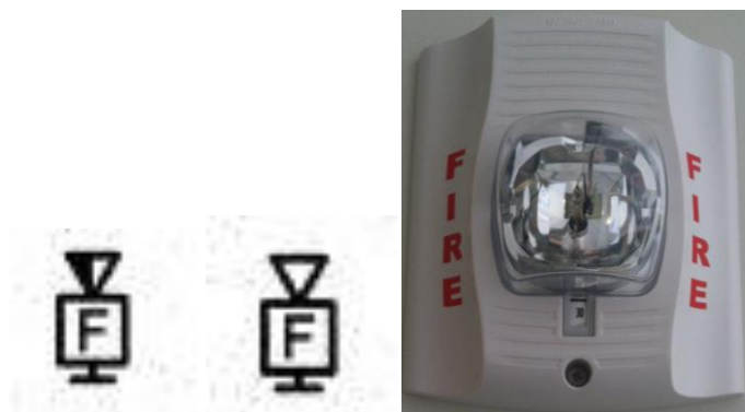
Figure 21 - Plan symbol of speaker/strobe, strobe and photo of strobe from building.
