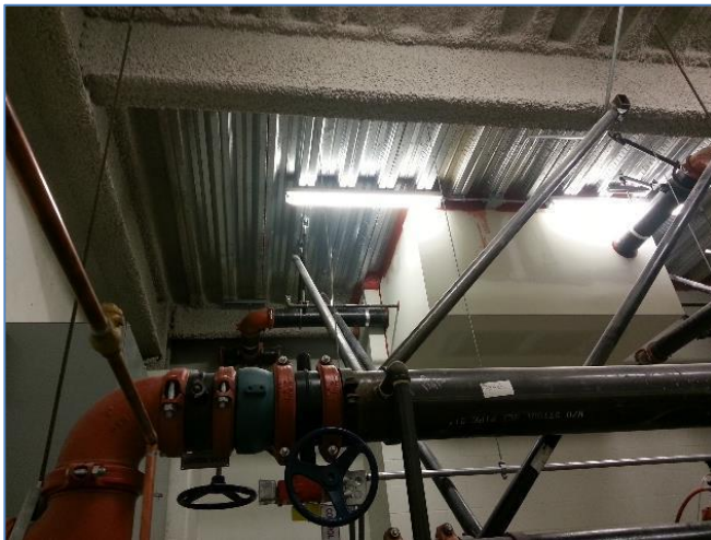
Figure 5 – Beam (left) and column (right) fire proofed with SFRM
