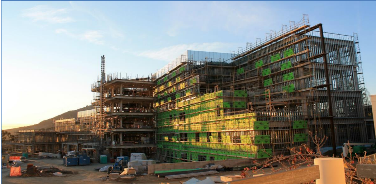
Figure 4 – CSM under construction
