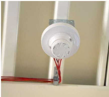
Figure 26 Harsh Condition Smoke Detector
