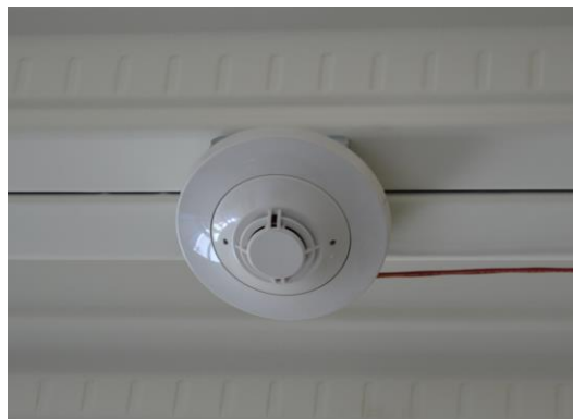
Figure 27 Multi-Sensor Smoke & Heat Detector
