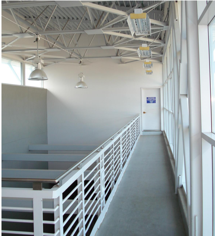
Figure 1-1. Third floor atrium and mechanical room
