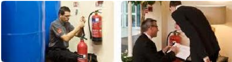
Figure 3.3: Fire extinguisher maintenance works
