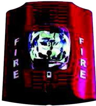
Figure 2.14: Typical Horn/Strobe installed in the Recreation Center
