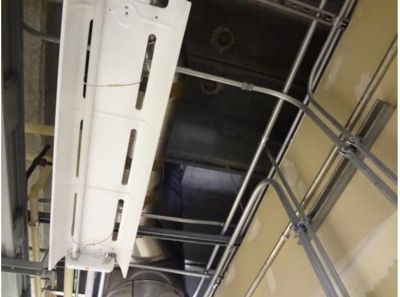
Second floor ceiling photo showing the floor slab of 3 rd floor
