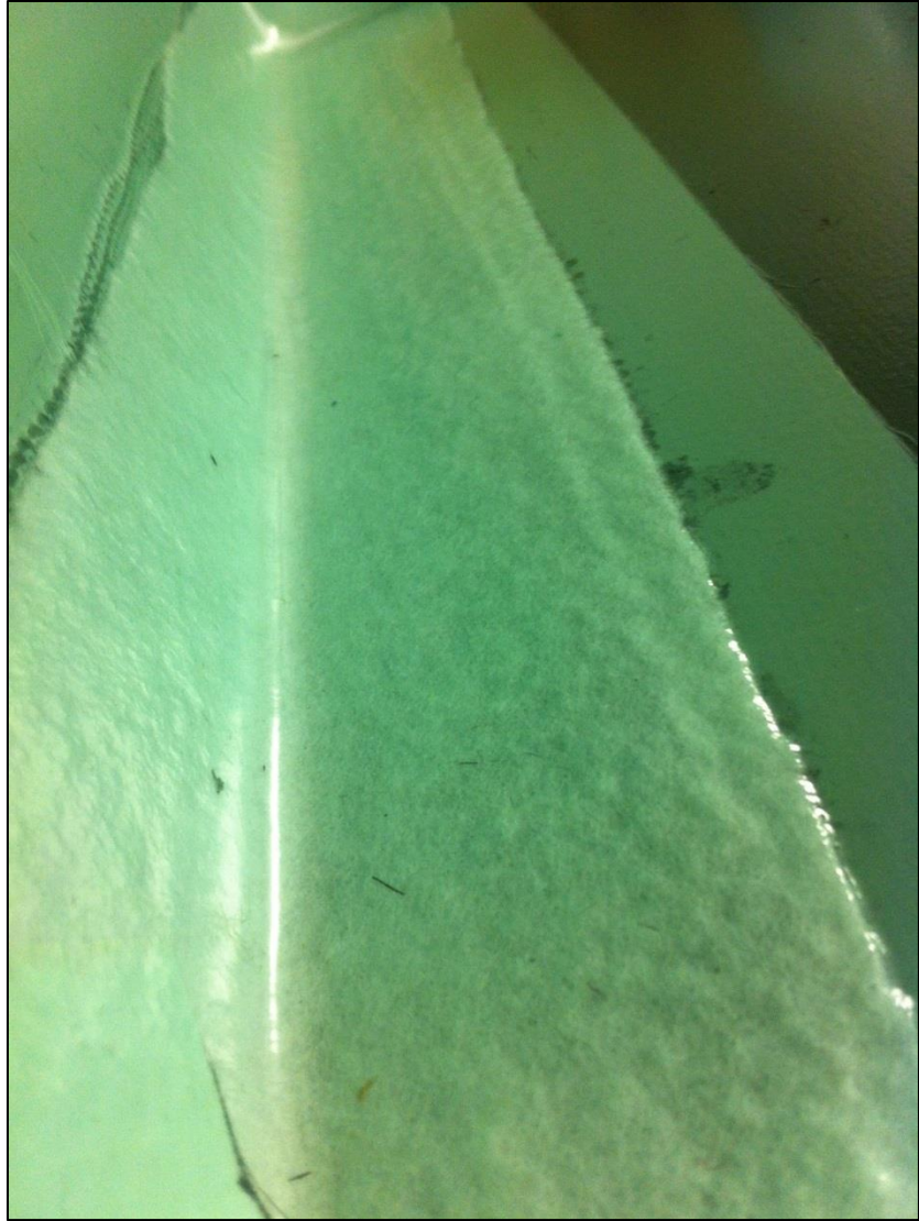
Figure 5.14: Close-up of a good vacuum on bend reinforcement.
