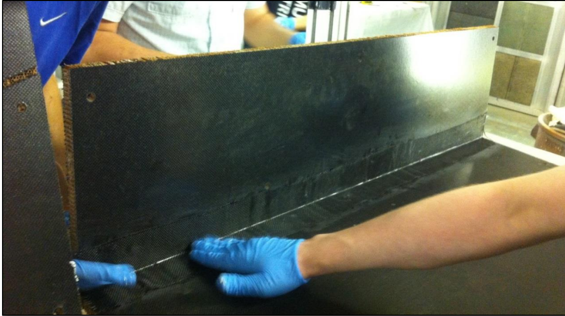
Figure 5.9: Smoothing wrinkles out of carbon tape. Tape has been laid up onto bend.
