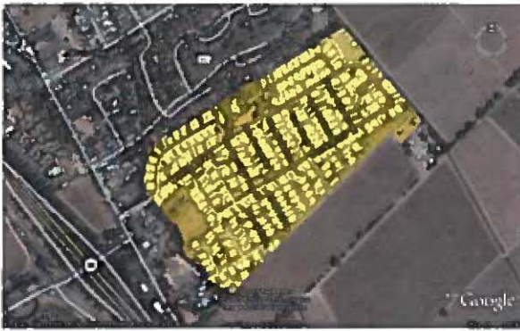
Fig. 1. Area protected by the flood barrier wall. Source: Google Earth™.
