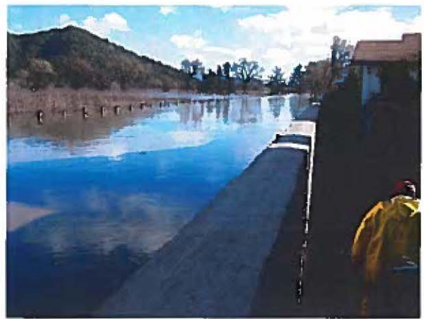
Fig. 3. Floodwaters at maximum height on the Yountville flood barrier wall, December 31, 2005. Source: City of Yountville.
