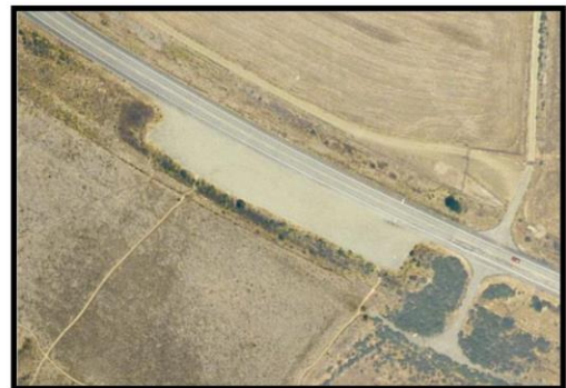
Location: PM 38.8 Size: ~60' X 440' spaces Visitor Amenities: None Ingress/egress: None Planned Improvements - Reduce in size and enhance
