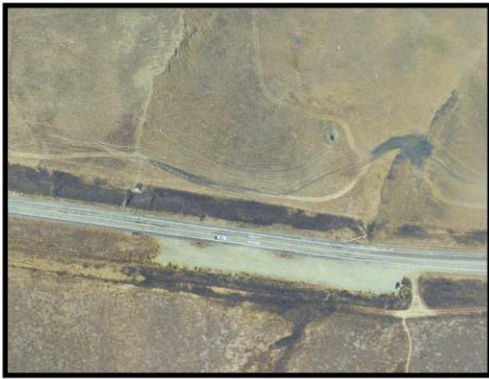
Location: PM 37.1 Size: ~50' X 480' spaces Visitor Amenities: None Ingress/egress: None Planned Improvements - Reduce in size and enhance
