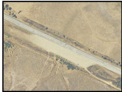
Location: PM 38.6 Size: ~50' X 340' spaces Visitor Amenities: None Ingress/egress: None Planned Improvements - Emergency Access only
