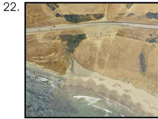
Location: PM 60.4 Size: ~.4 Acres Visitor Amenities: None Ingress/egress: None Planned Improvements CCT access
