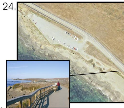
Location: S. Elephant Seal (PM 62.7) Size: ~50 spaces Visitor Amenities: boardwalk, Interpretive signage/kiosk, benches Ingress/egress: Left-turn Channelization (500'), 8' right hand shoulders
