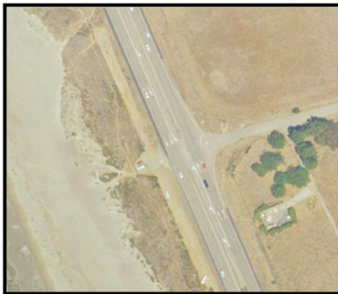
Location: PM 32.75 Size: ~40 spaces Visitor Amenities: None Ingress/egress: 230' left-turn lane, 8 foot shoulders Planned Improvements: - Reduce in size and enhance
