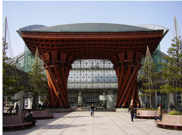
Figure 16 - Kanazawa Station Main Entrance (Photo Credit: Adam Kahava; Source: "Train Stations", 2014)
