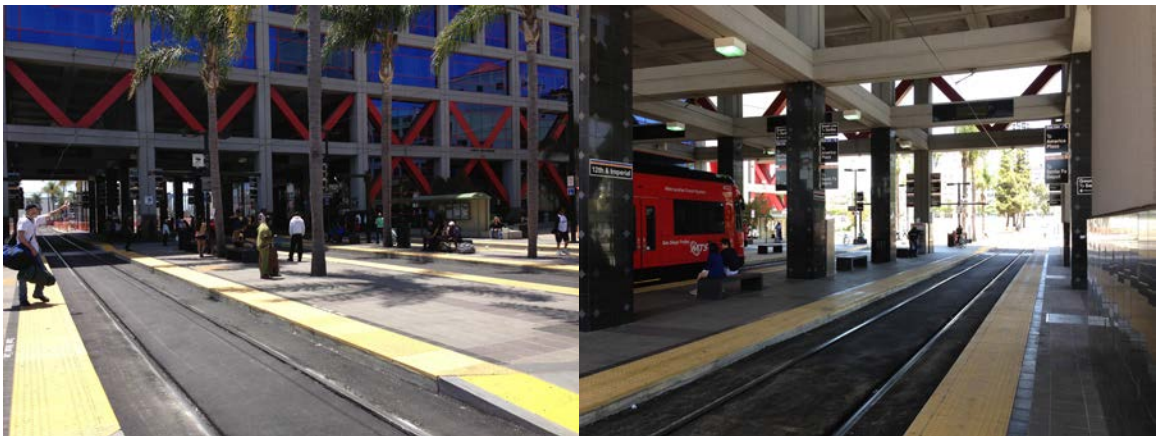
Figure 25 - 12th and Imperial Transit Center, Exterior Plaza (Photo Credit: Derek Holloway)
