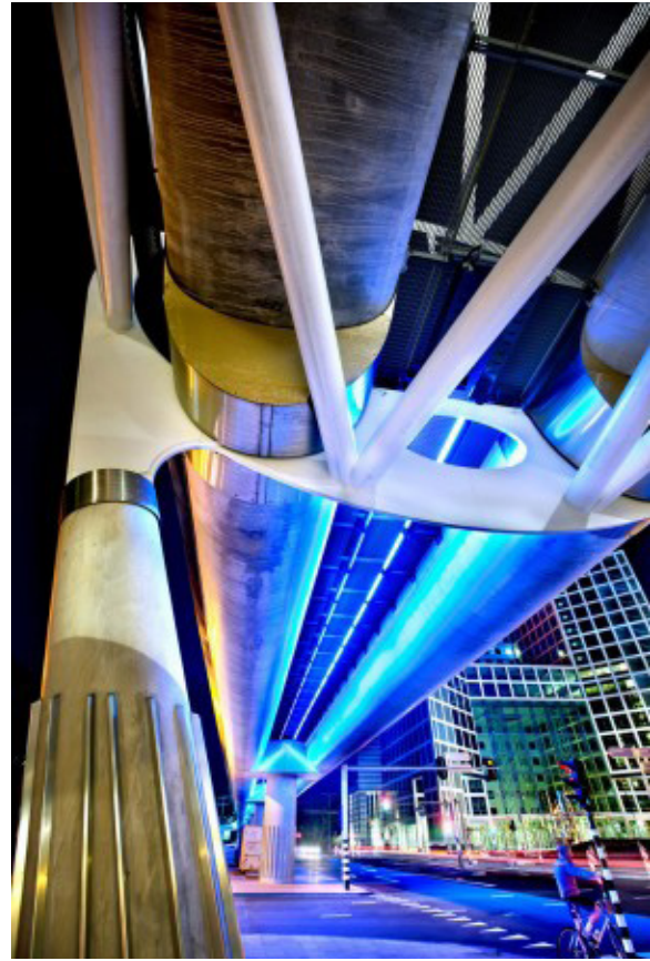
Figure 7 - Station Lighting (Source: RandstadRail, 2009)
