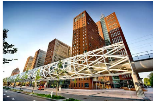
Figure 6 - Street View of Elevated Space-Frame (Source: RandstadRail, 2009)
