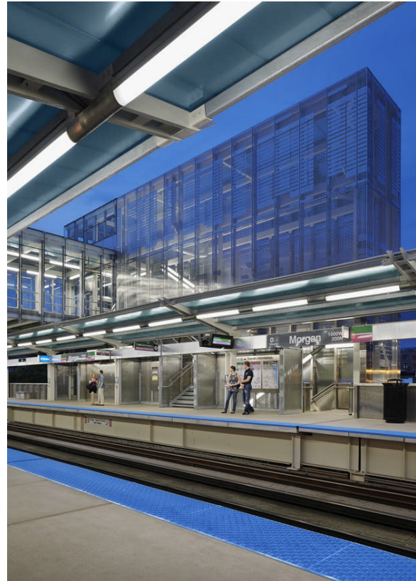
Figure 9 - Elevated Platform and Tower (Photo Credit: Kate Joyce Studios; Source: Gerfen, 2013)
