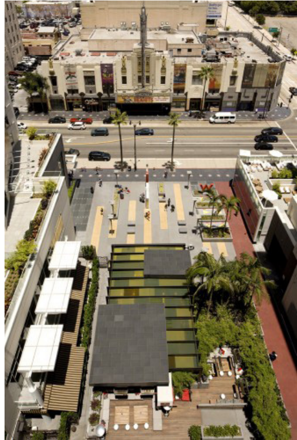
Figure 4 - Hollywood and Vine Station Entrance and Plaza (Photo Credit: Tom Bonner; Source: “Hollywood and Vine Metro Portal and Plaza”, 2013)
