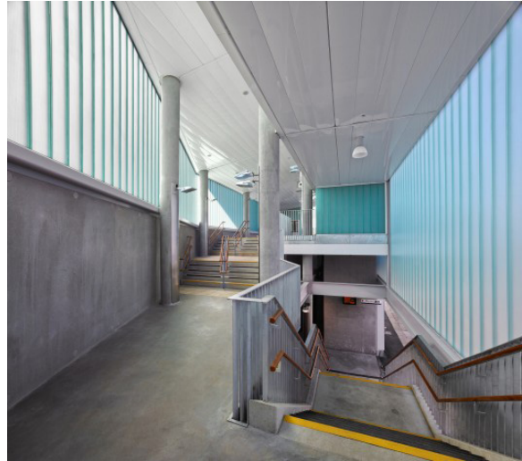
Figure 23 - Interior Corridor Between Main Entrance and Platform (Source: “Dalmarnock Station”, 2013)
