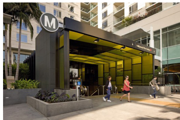
Figure 32 - Main Entrance to Subterranean Station (Photo Credit: Tom Bonner; "Hollywood and Vine Metro Portal and Plaza", 2013)
