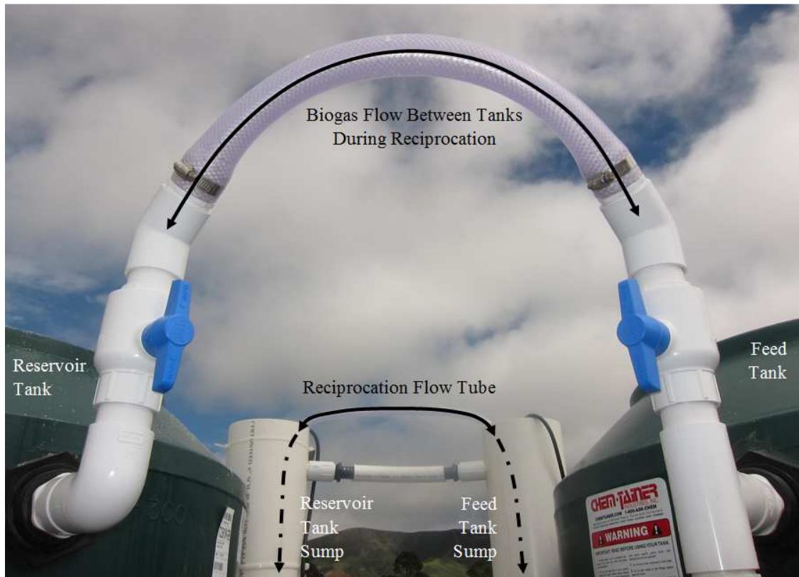
Figure 3.6: Configuration for reciprocation between tanks. Liquid levels were raised and lowered within the two tanks as flush water was pumped from one tank to the other and then back. Biogas was also distributed between tanks to account for displaced liquid volumes caused by reciprocation and keep digester system pressures relatively constant. Submersible pumps were located inside and near the floor of the sumps. Photo taken before attachment of silver insulation around green tanks.
