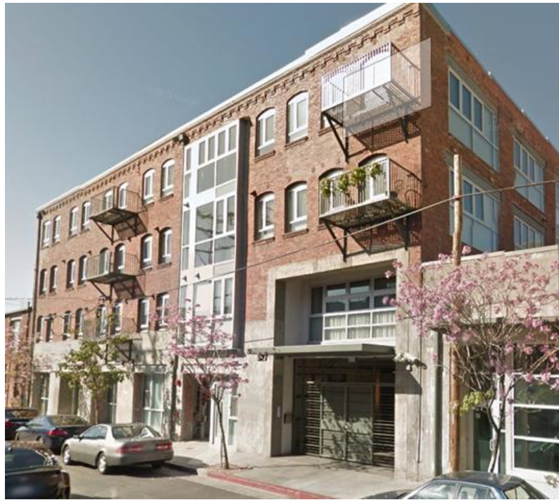
Figure 16: View of Barker Block Warehouse (Google Maps, 2014)
