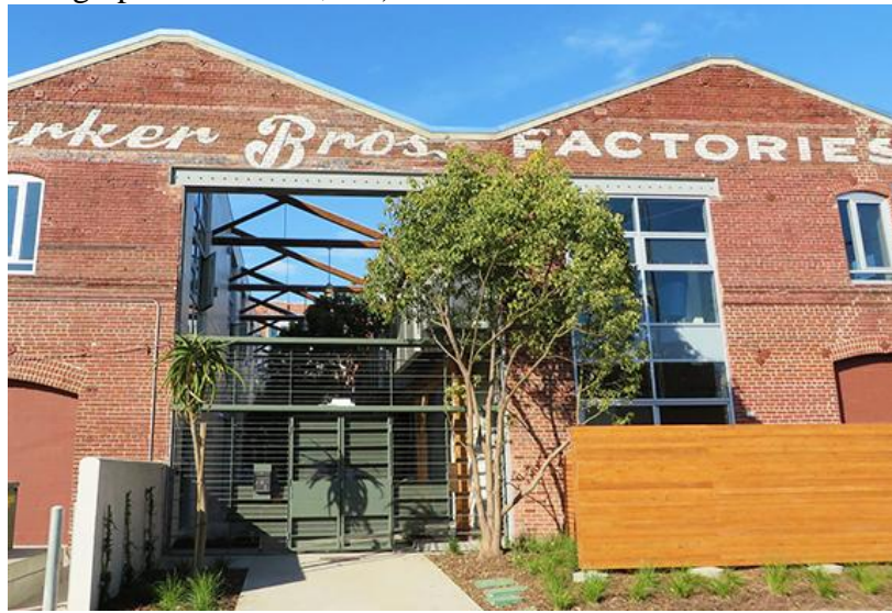
Figure 15: Primary facade of Barker Block Warehouse No.1 (Photographer unknown, n.d)
