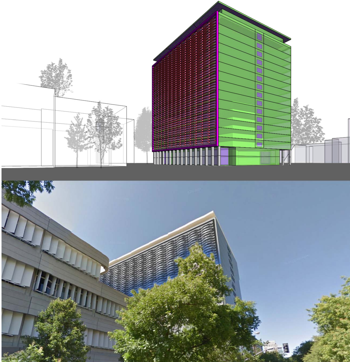
Figure 5.2.4: Egg-Crate Shade Device Perspective
