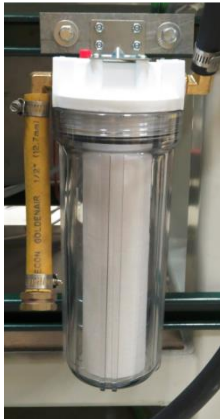
Figure 10. 20 Micron water filtration unit
