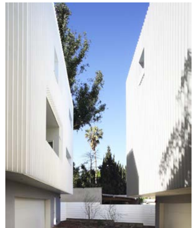
While the homes are configured to provide adequate access to the garages for cars, the interior spaces are arranged so that windows and balconies do not directly face each other. This creates a better sense of privacy for homes that are closely spaced.
