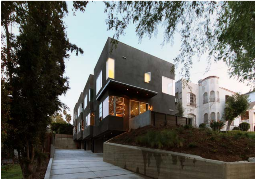
The slightly sloping site resulted in the units having a “stacked” configuration and the garages being cut into the slope. A 35 foot front setback was provided
