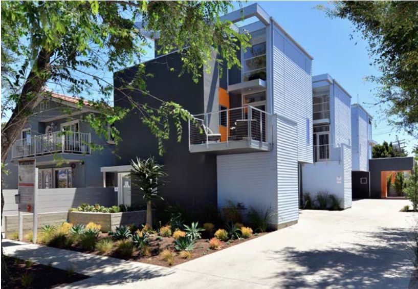
The Cullen Street development demonstrates a side access driveway with the front unit having a strong relationship to the street.
