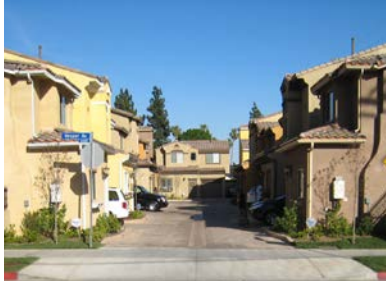
Enhanced paving denotes the entryway to the Vesper Village development in Van Nuys.
