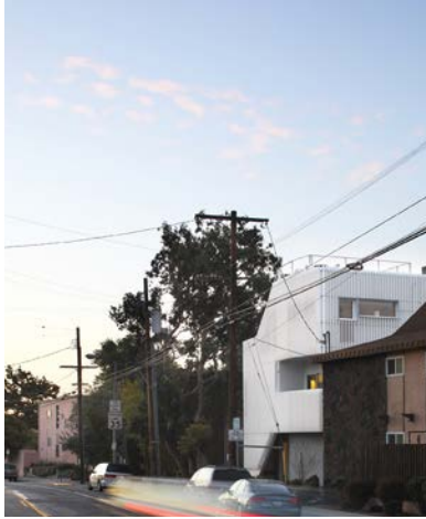
The Buzz Court development alternates texture, color, and materials on the front facade.
