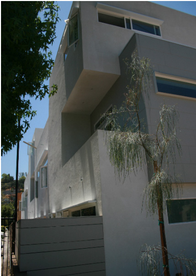
Sensitive window and balcony placement in the Rock Row development are key to enhancing the light and ventilation of the home's interior.
