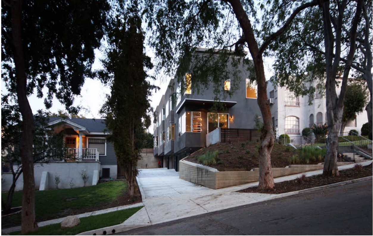
The site has a two story building on one side and a single story residence on the other. As a result, the mass and height of the buildings are located on the side adjacent to the two story building.
