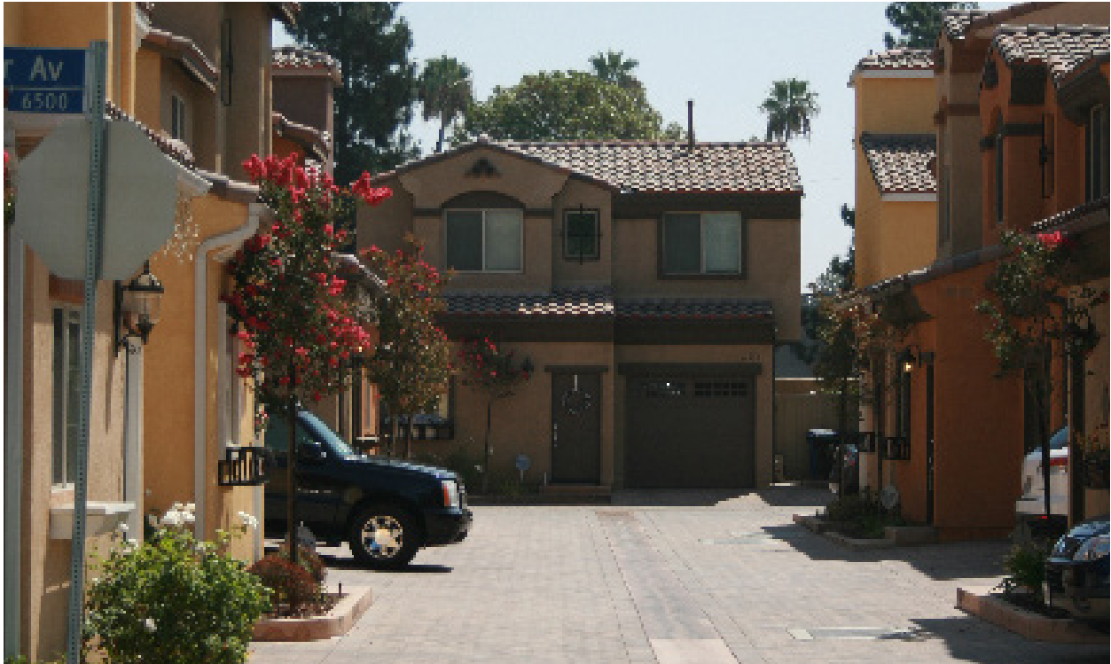
The 26-foot width between homes is syncopated with a 32' distance occurring at the garage/parking. This articulates the massing of the buildings and prevent the pedestrian from feeling "boxed in".
