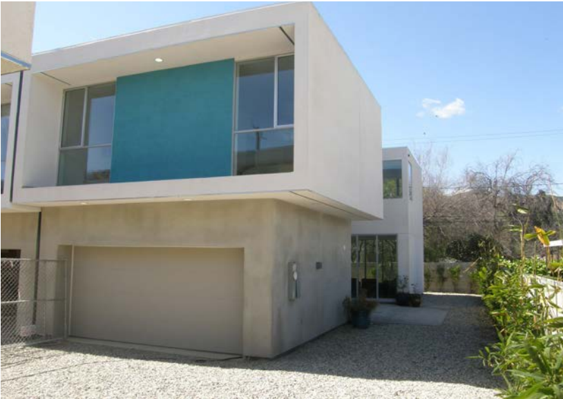
This home on one of the edges of the project shows the interior courtyard space connected to a side yard, providing additional usable open space.
