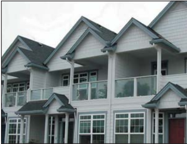
Excessively varied and multi-pitched roofs risk create visual chaos.
