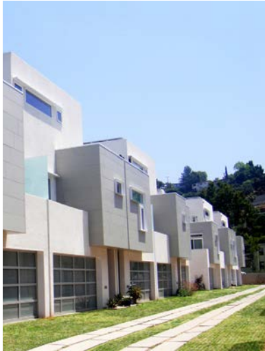
The Rock Row development in Eagle Rock features a central driveway with alternative paving.
