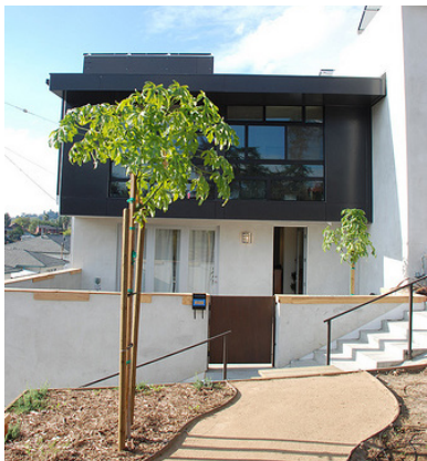
Permeable paving (decomposed granite) allows the infiltration of storm water. Homes feature private patios.
