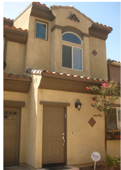
Open sight lines to front doors.
