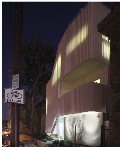
The facade treatment provides for a visually interesting and appealing display at night. The shading element provides privacy for the residents while still allowing light to be displayed along the sidewalk. The front entrance is clearly illuminated for safety and delineation.
