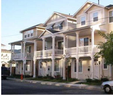
Sufficient space should be provided for an entry, landing and transitional landscaping between the sidewalk and private entryway.
