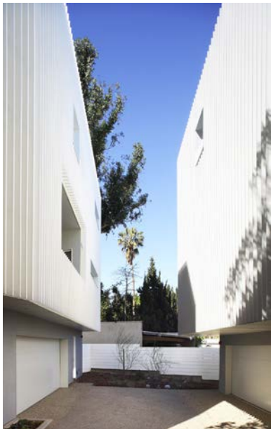
Small lot homes must be structurally independent with no shared foundations or common walls.
