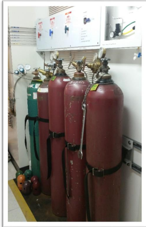
Figure 3.35 Gas Tanks Need for Sputtering Process
