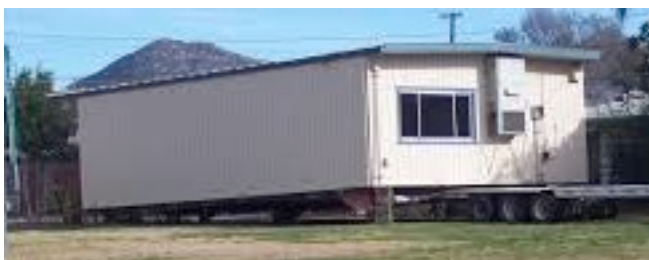
Figure 4. Portable Classrooms have individual HVAC equipment that is widely criticized as unhealthy, wasteful and noisy.
