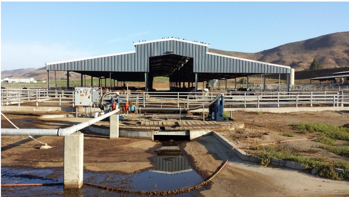
Figure 4. The Cal Poly Dairy Unit cattle freestall barn.
