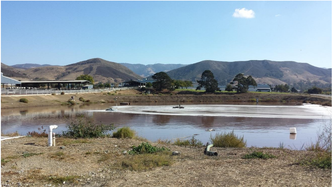
Figure 6. The aerated dairy lagoon at Cal Poly.
