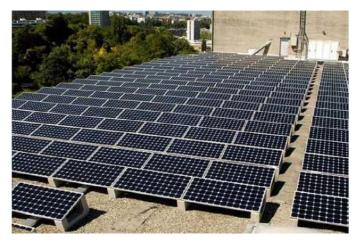
20 Kilowatts of Solar PV amounts to about 110 185w 24v solar PV panels. For a typical roof mounted installation, about 1,240 square feet or 115 square meters would be required for these 110 solar panels.
