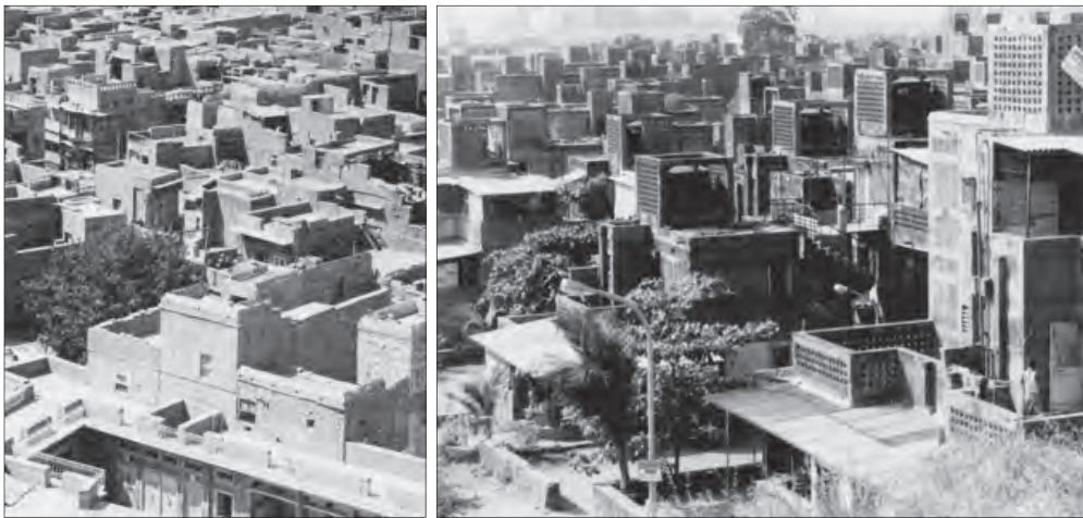
Figure 7: The Income Tax Colony, Navi Mumbai: the precedent Jaisalmer, Rajasthan (left) and the design (right), Raj Rawal, architect, 1996+. (photos by the author)
