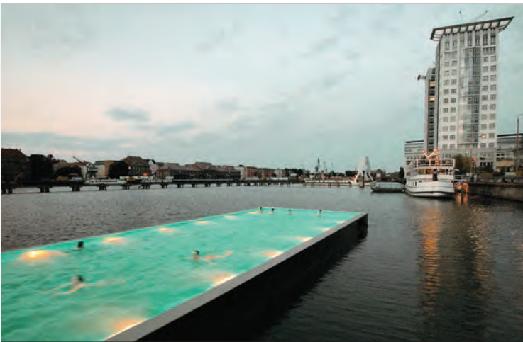
Figure 7: Berlin's floating pool: comfortable swimming is offered the entire year at the river level; roofless in the summer and covered during winter. (photo by AMP Architects, S. Lorenz and G. Wilk)
