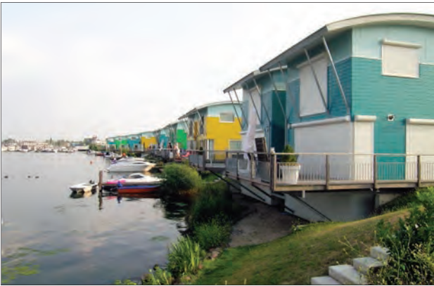
Figure 5: Netherland's Maas amphibious houses: located on firm soil, they are anchored to the site by a vertical structure and are prepared to float during a flood event. (photo: Factor Architecten and Dura Vermeer)
