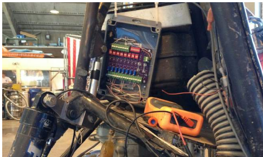
Figure 53. Rear Link Amplifier Offset Calibration Process (On-Car)
