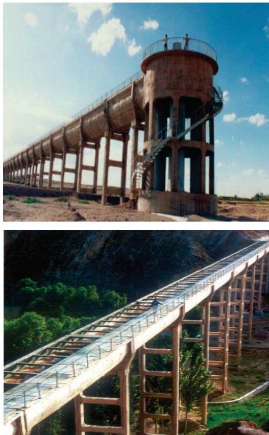
Figure 3 Structure of 5#U-type aqueduct in Jingdian Irrigation District
