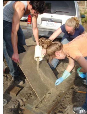
Figure 8: Placement of sand in cavity of double wythe wall
