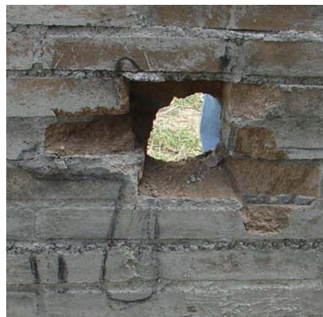
Figure 14: Double wythe wall and penetration, back face
