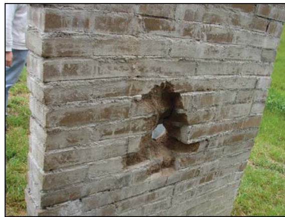
Figure 10: Single wythe wall and penetration, back face
