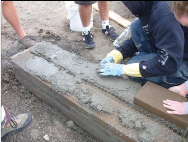
Figure 7: Chicken wire used to tie double wythe wall together.
