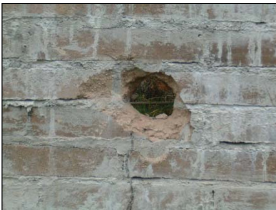
Figure 9: Single wythe wall and penetration, front face
