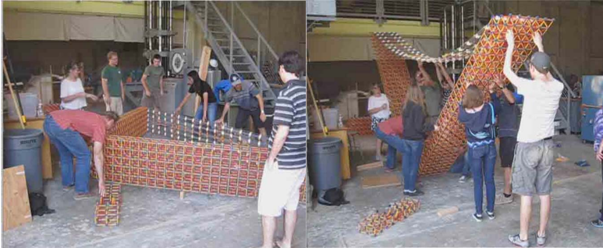
Figure 11: Students encountered new challenges when constructing and erecting the sub-assemblies.
