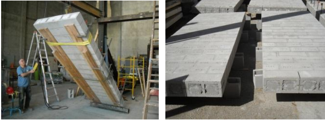
Figure 9: (a) Lowering the Wall and (b) Lowered Walls
