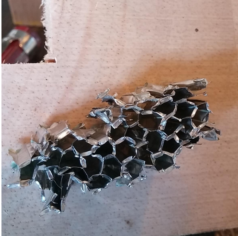
Figure S3. A sample of the failed core shows the results of continued out of plane loading after the core sheared loose inside the sandwich structure (shown later).
