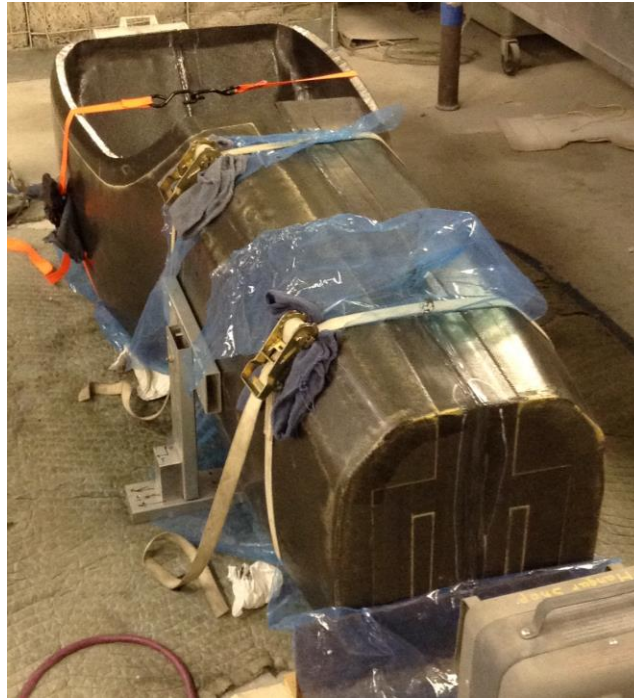
Figure 49. The monocoque while the resin slurry is curing. Note how FEP was placed between the monocoque and ratchet straps to prevent unwanted bonding.
