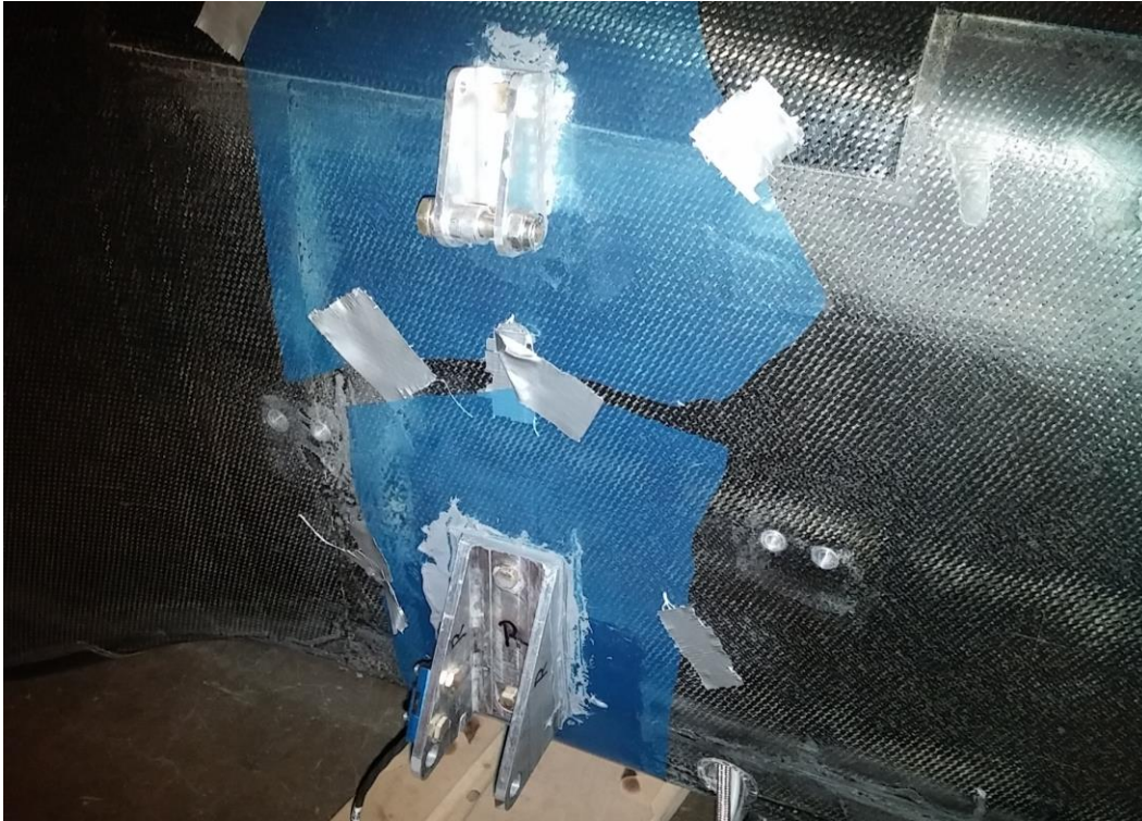
Figure 59. Structural aluminum putty was used to create a matching surface for the upper and lower suspension mounts. FEP was used to keep the adjacent areas clean during the process.
