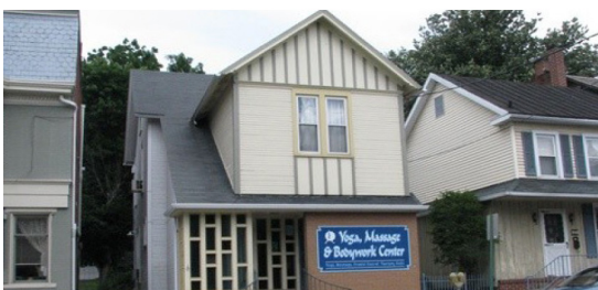
Figure 9: Facade improvements in downtown Lewistown – Top: before, bottom: after Source: http://www.nado.org/vibrant-rural-ommunities-lewistown-pennsylvania/
