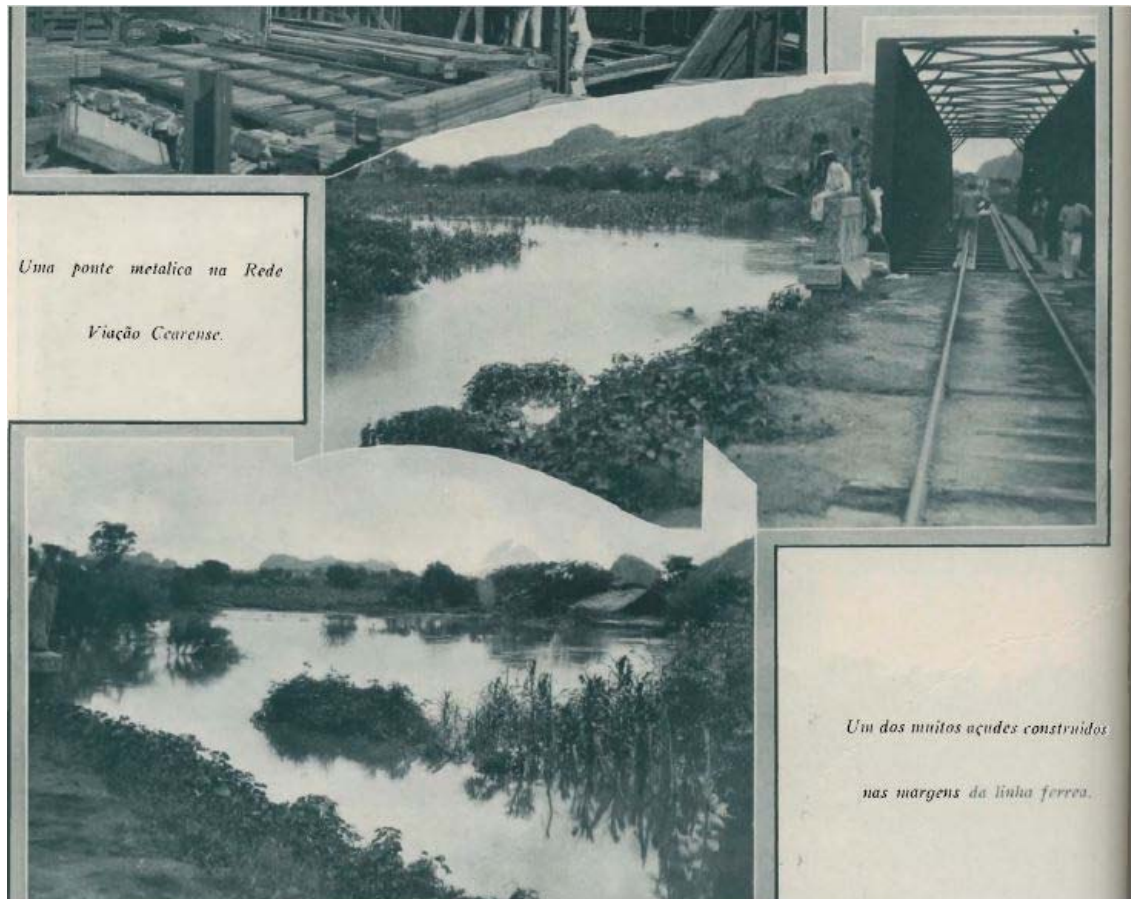
Figure 17- Railroad of the Ceará State, built by IFOCS
