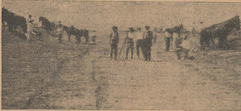
Surveyors and excavators working on main irrigation canal.
