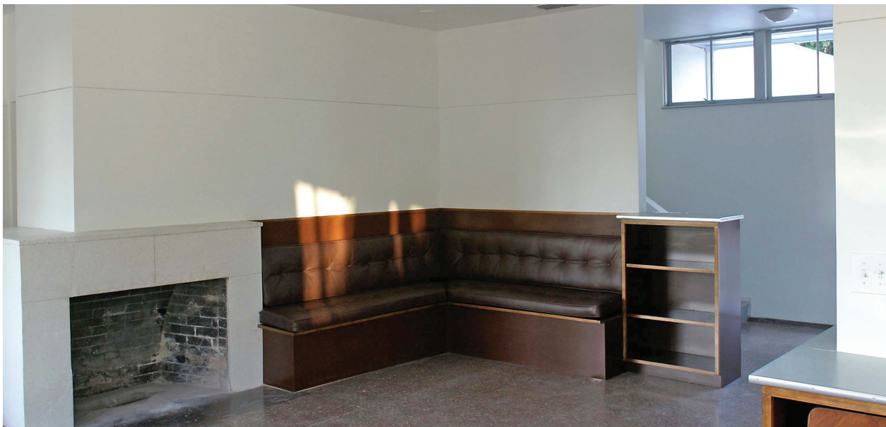
Fireplace and living room ( after )
