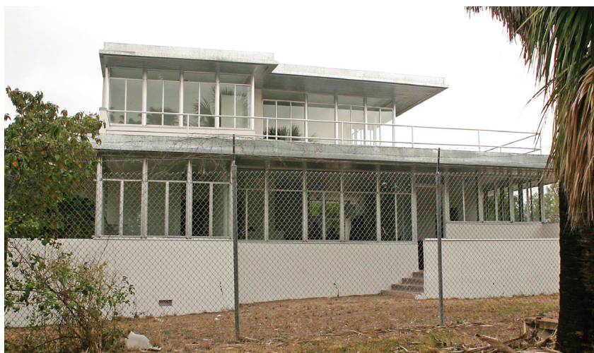
Nearing completion (early 2008)
