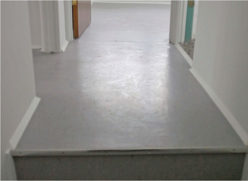
Second floor hall (after)
