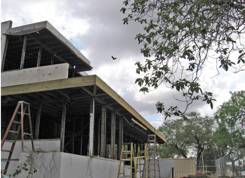
Southwest corner (during)
