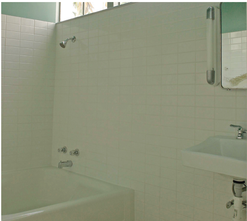
Upstairs bathroom (after)
