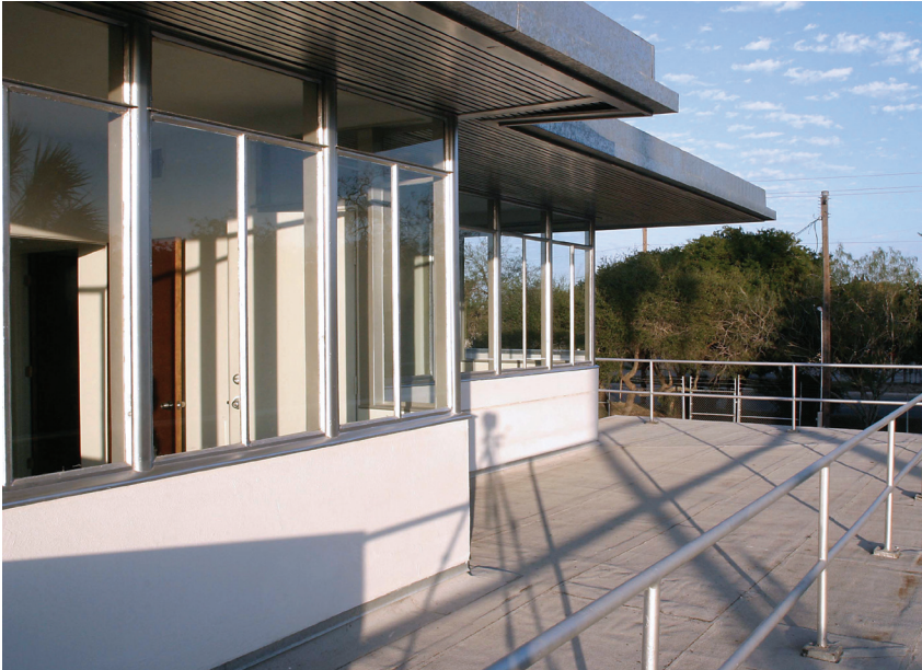
Roof deck (after)
